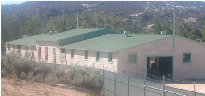
One of the Camp Lockett stable buildings purchased by MTM. Roof repair has been completed and window and door repair is in progress.
